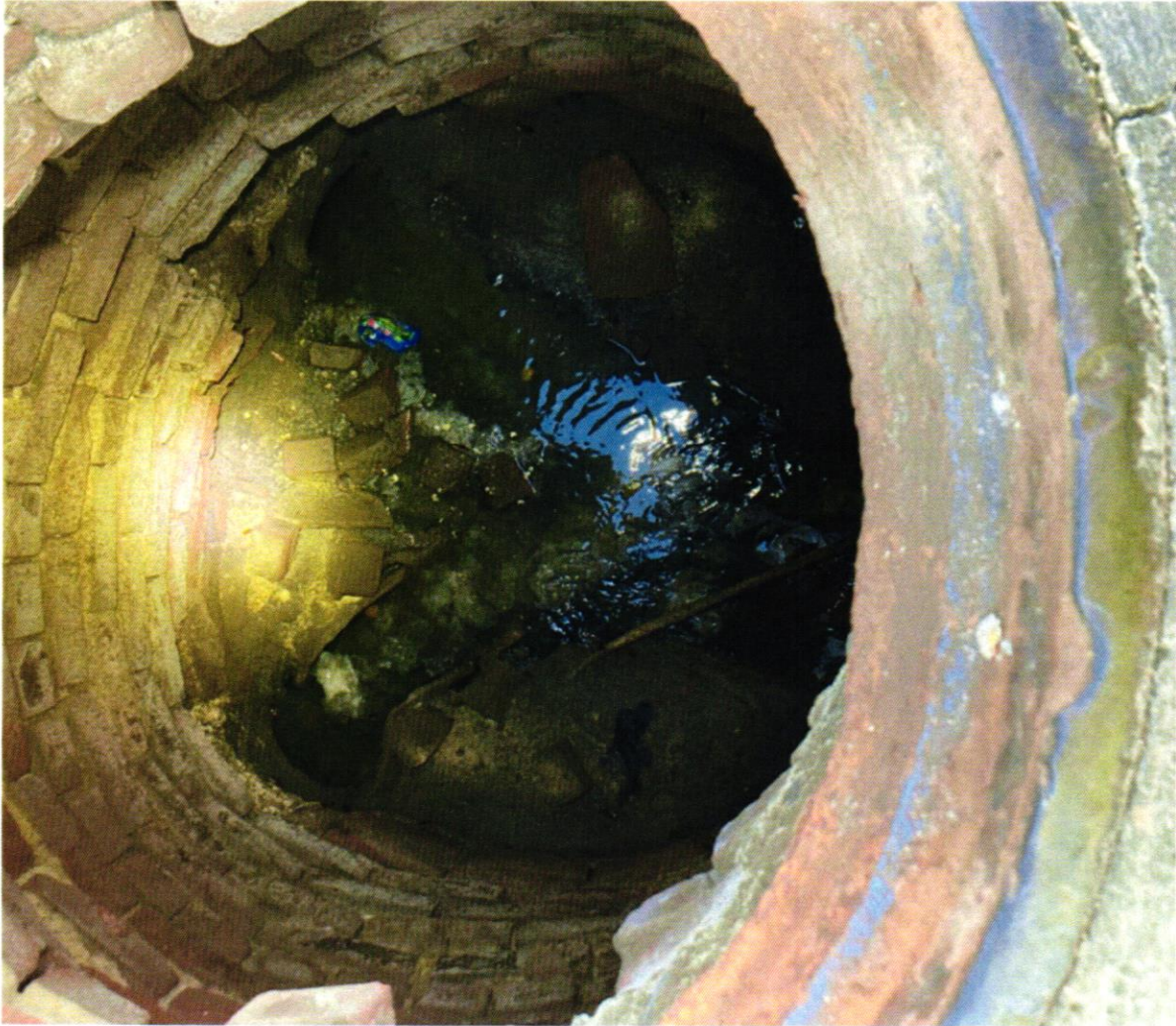
View within MH #54 to be rehabilitated.
