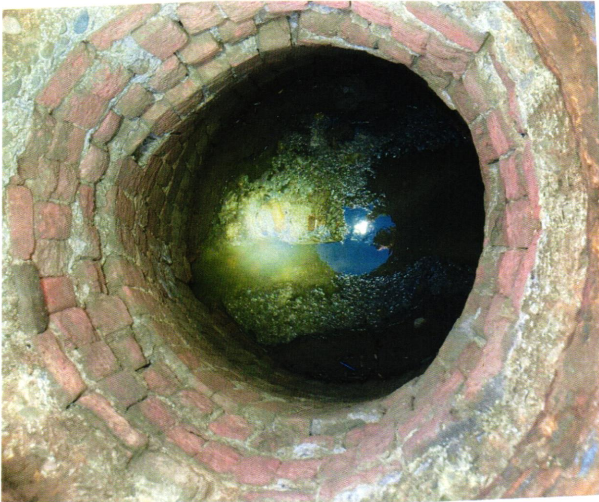
View within MH #56 to be rehabilitated.
