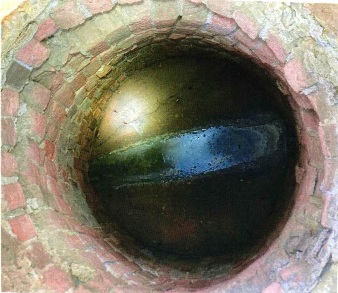
View within MH #55 to be rehabilitated.
