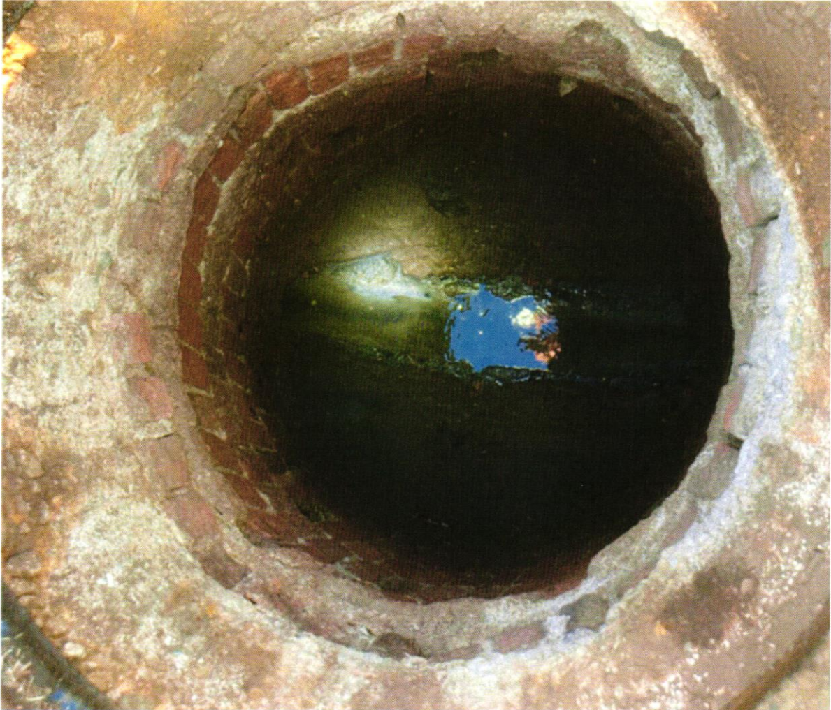
View within MH #58 to be rehabilitated.
