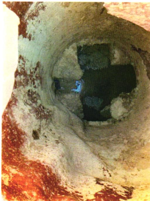
View within MH #1142 to be rehabilitated.
