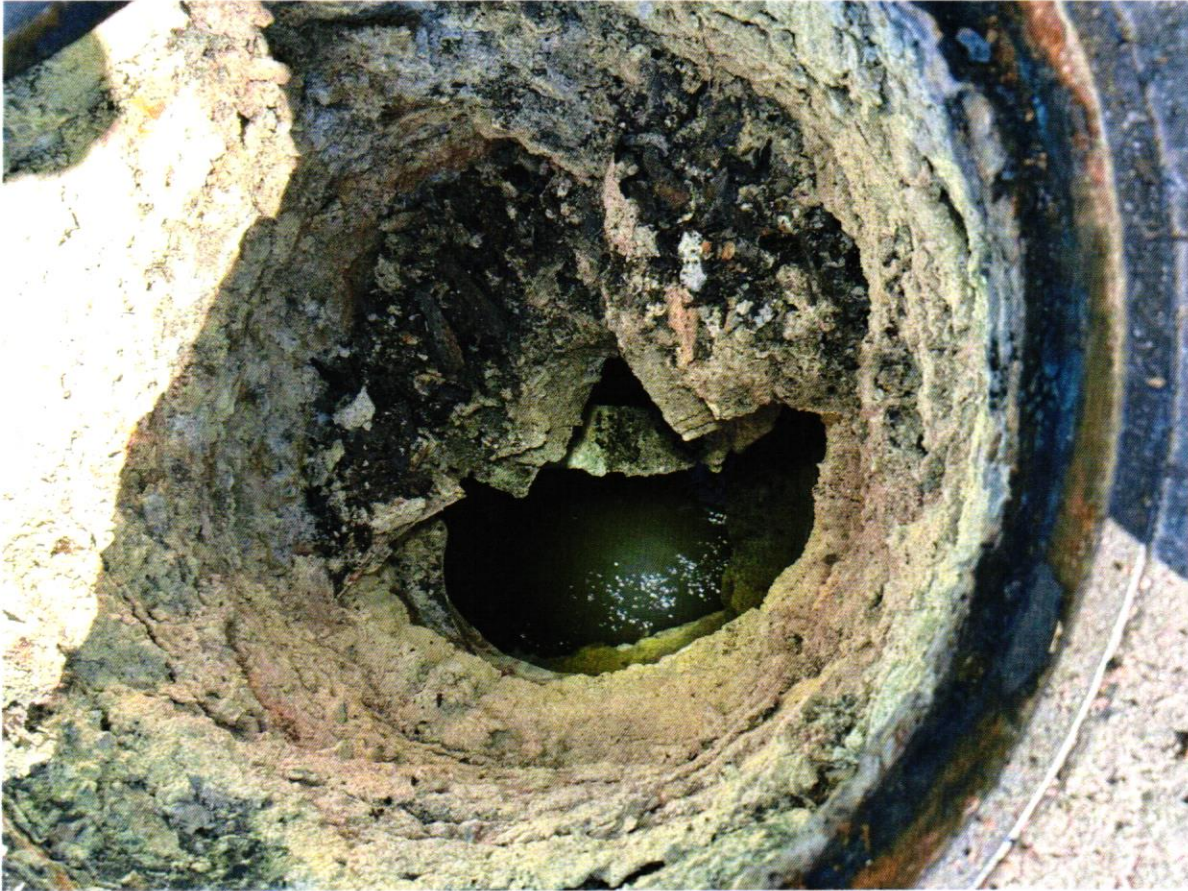
View within MH #348 to be rehabilitated.
