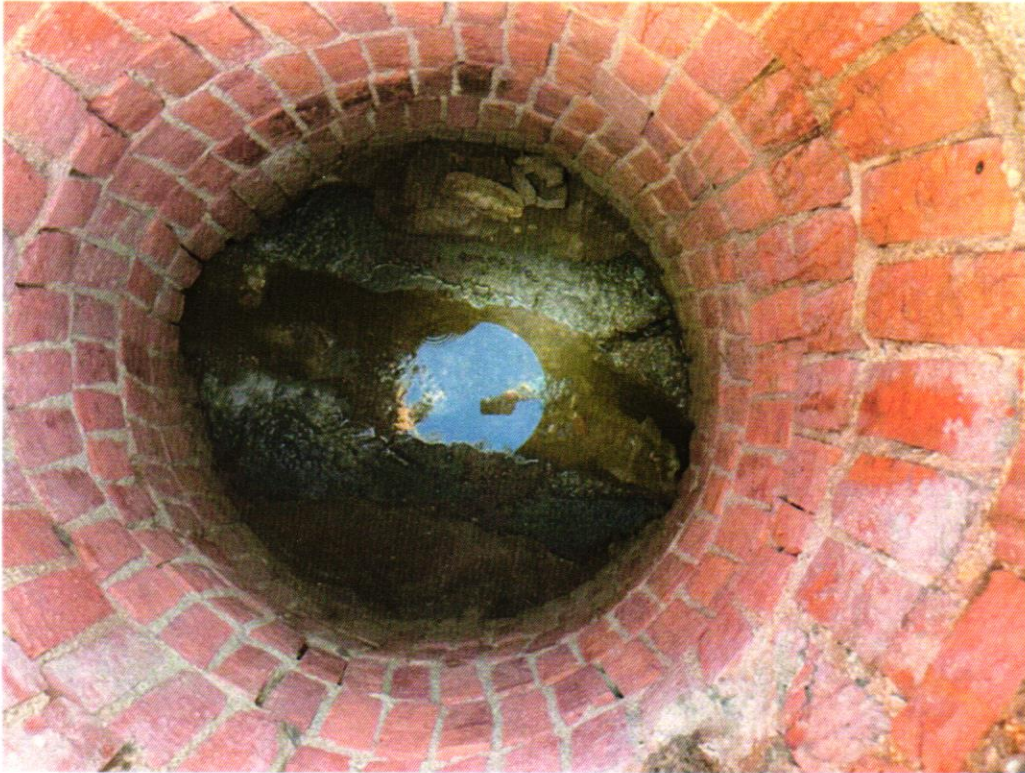
View within MH #42 to be rehabilitated.
