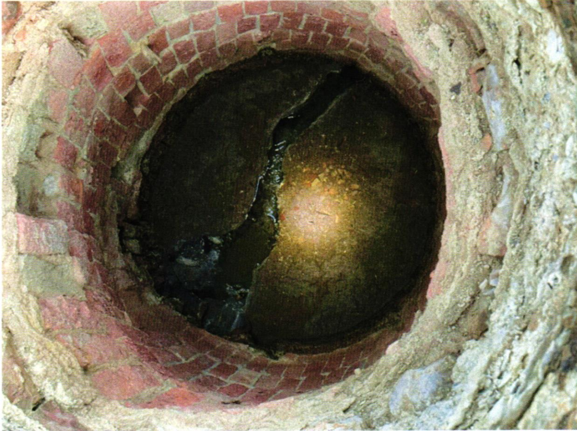
View within MH #51 to be rehabilitated.
