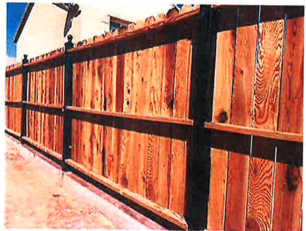
Ornamental Iron and Wood Fence
