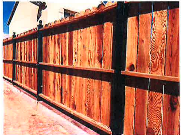
Ornamental Iron and Wood Fence
