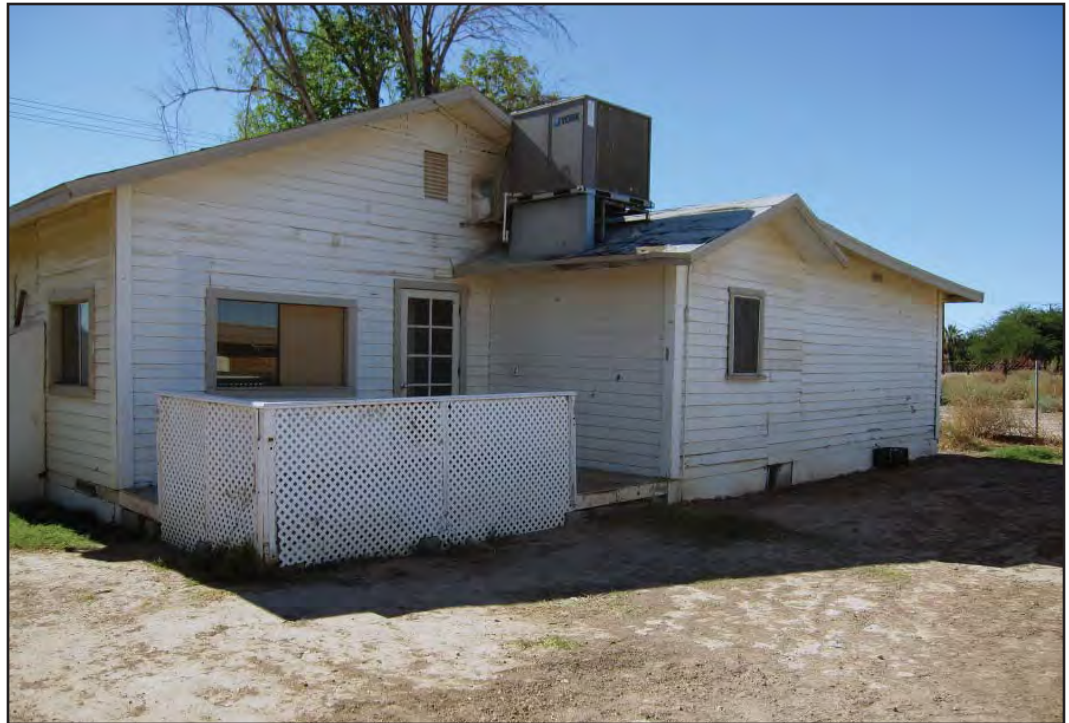
PHOTOGRAPH 9 Rear (North) Façade of the House
