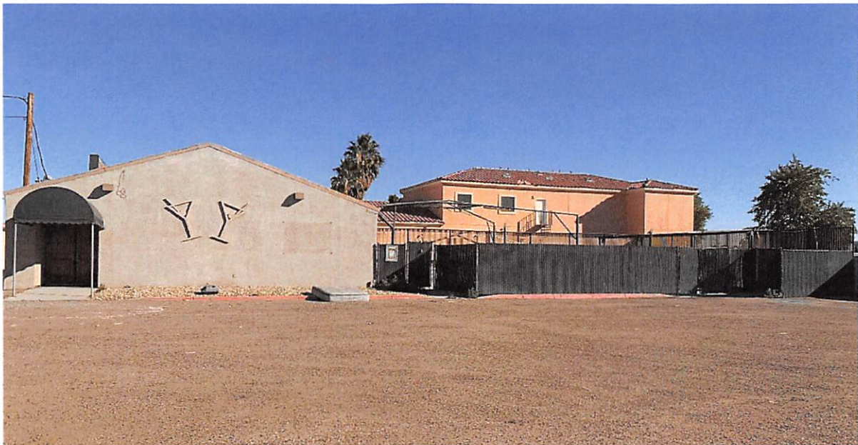
BACK VIEW OF ENTRANCE AND PATIO
