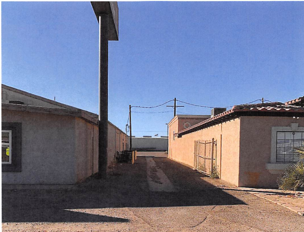
FRONT EAST ENTRANCE
