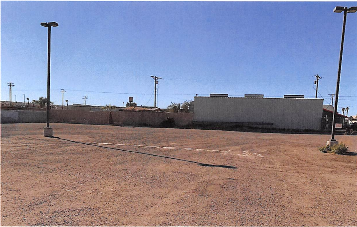
PARKING LOT AND LIGHTING
